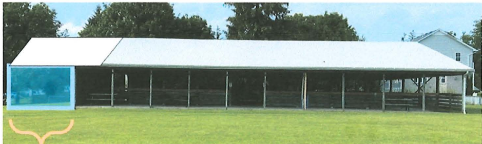
Extend the Ag Pavilion 20' to the west: 20' concrete pad and extending the roof 20', maintaining the current roofline
