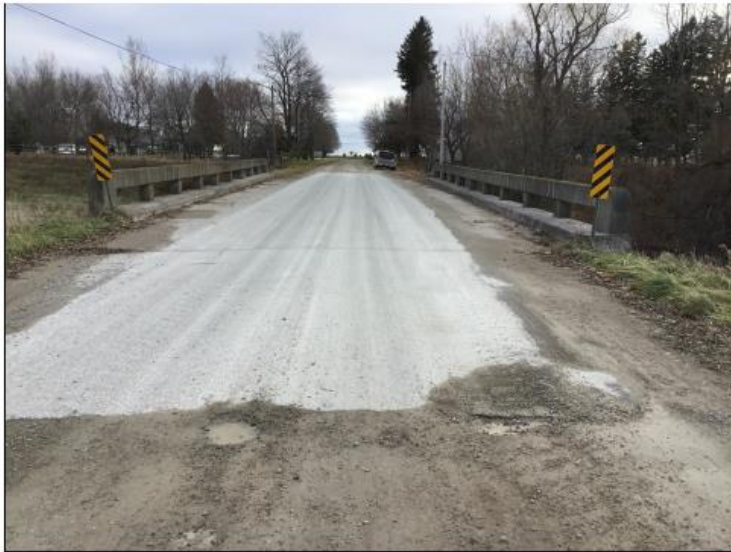
Description: North Approach (looking south)
