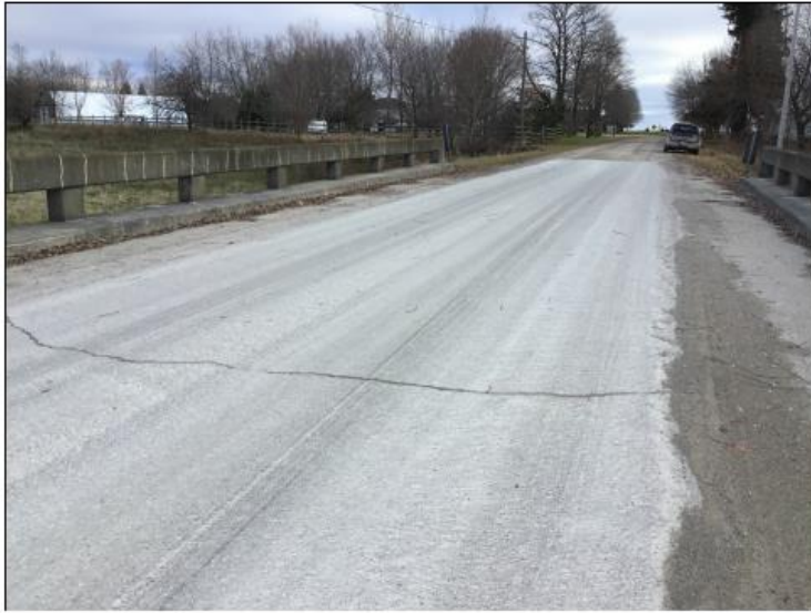
Description: Wearing Surface (looking south)
