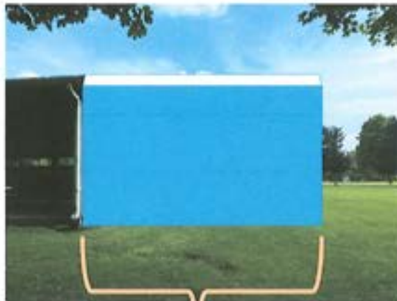
20' enclosed addition on the north half
