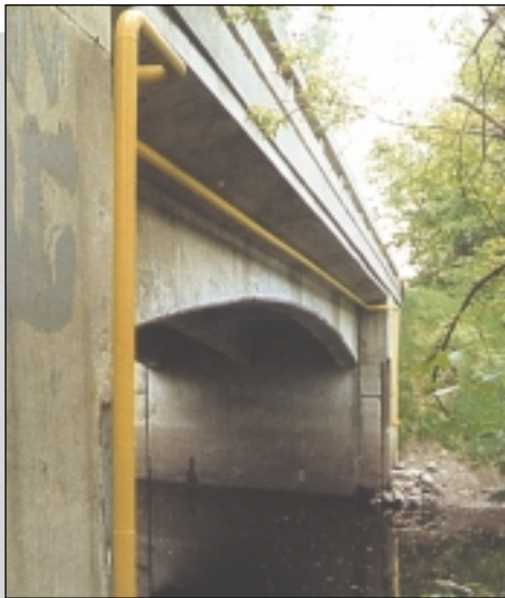
Attaching gas line on a bridge.
